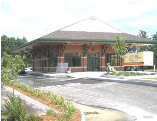
New intermodal terminal at Exit 2 in Salem
