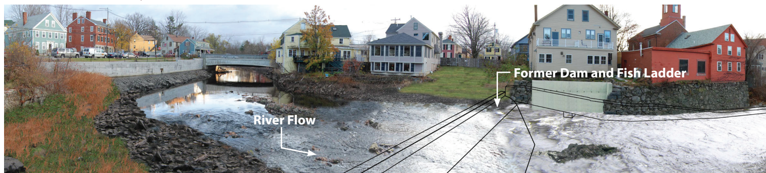
Proposed dam removal photomontage | This image was developed using hydraulic engineering and digital photography tools, and depicts what the river in the vicinity of the dam would most likely look like under normal flow conditions if the dam were to be removed.
