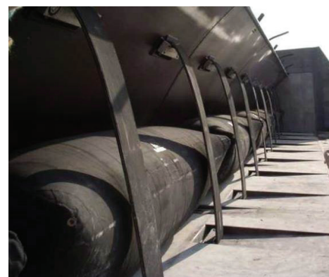
An example of an inflatable Flashboard/Gate system, similar to Alternative H.
