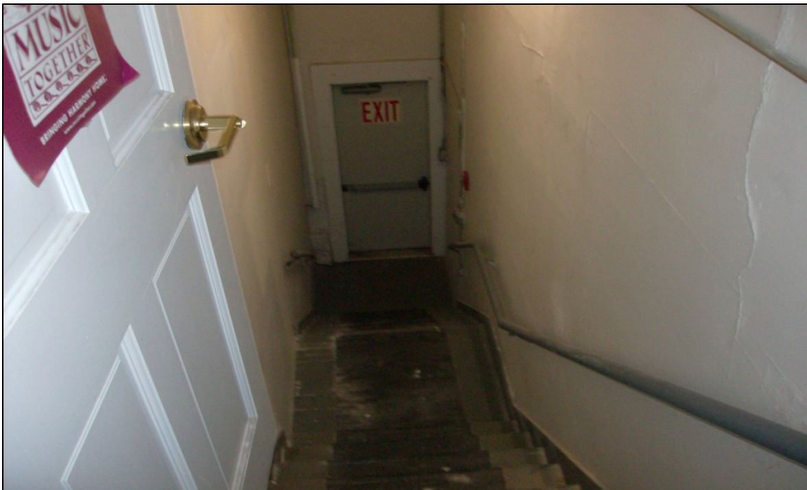
Emergency exit stairs from the second floor.
