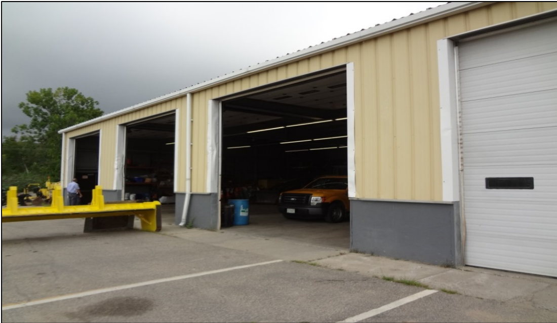
DPW Garage looking west at four truck bays.
