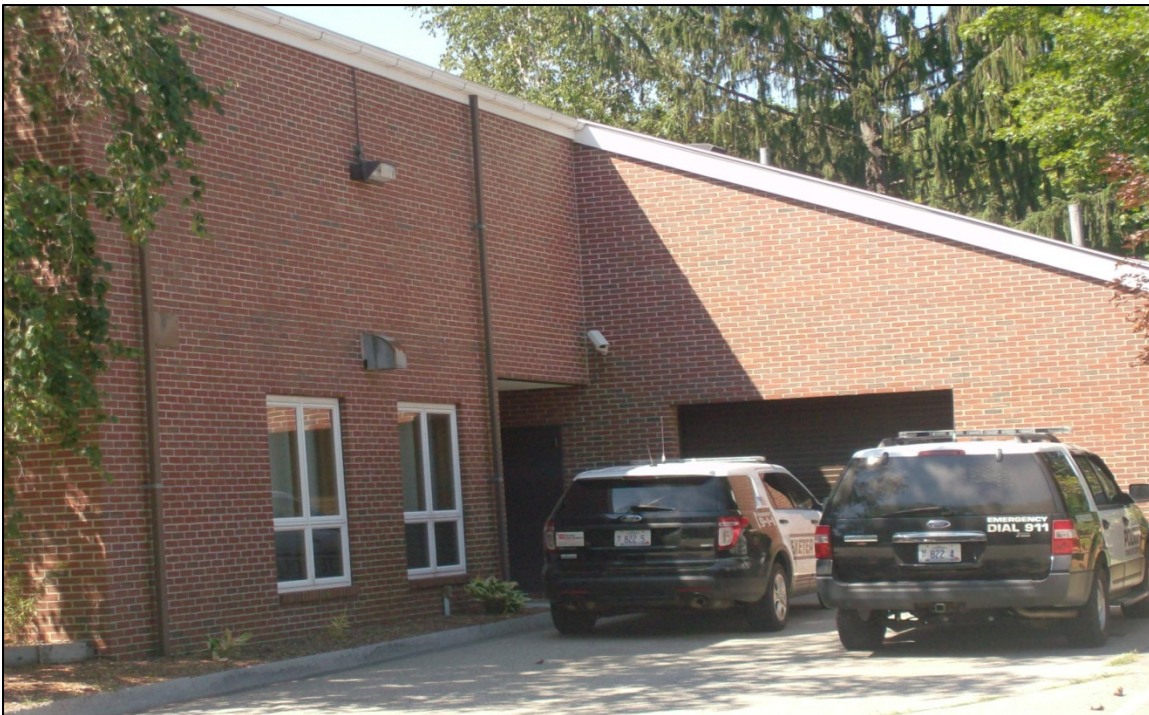
Police sally port on east side of building.
