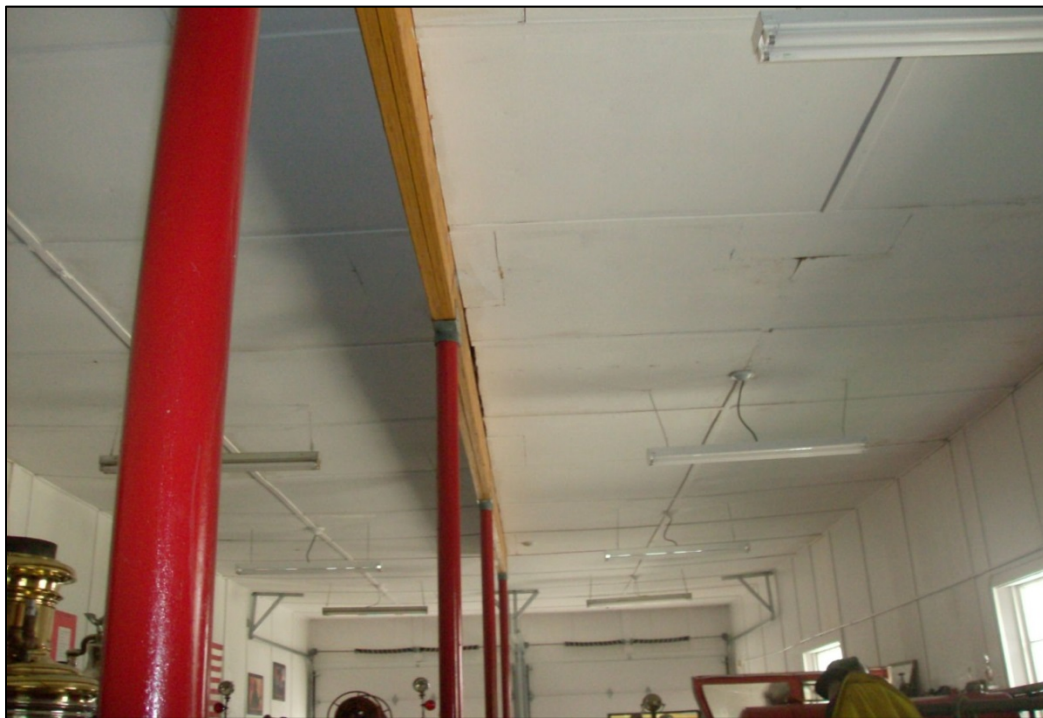
New laminated beam and post added to support ceiling in Fire Museum.
