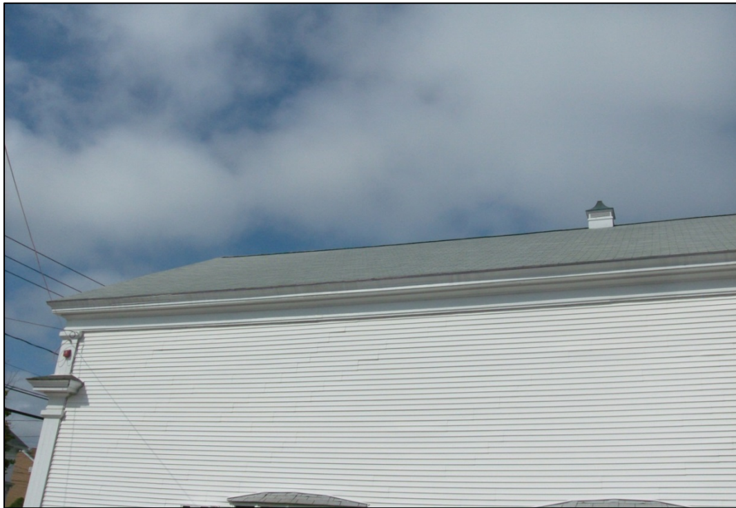
Roof of Senior Center. Shingles in good condition.
