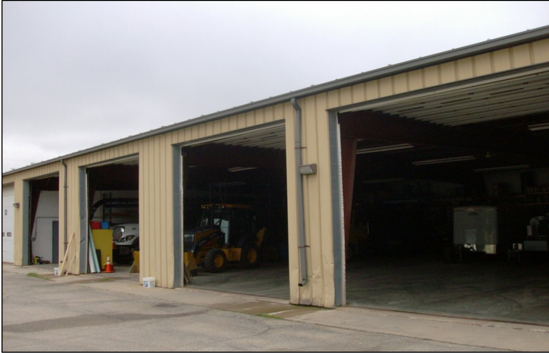
Front of Water Department Garage.
