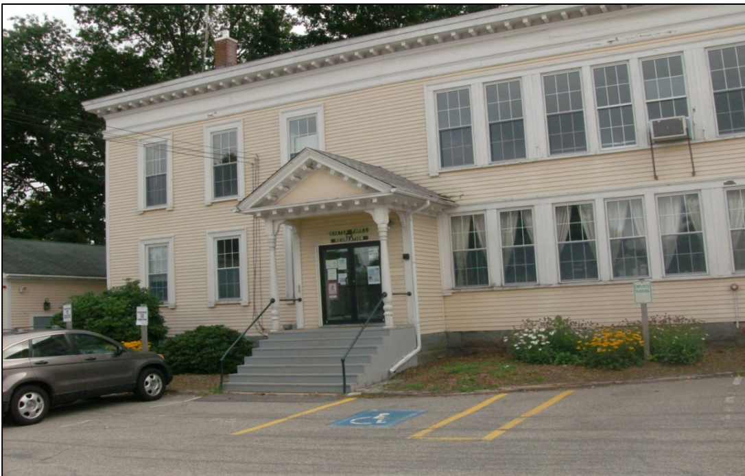
Main entrance from parking lot. Note handicap parking, but entrance is not accessible.
