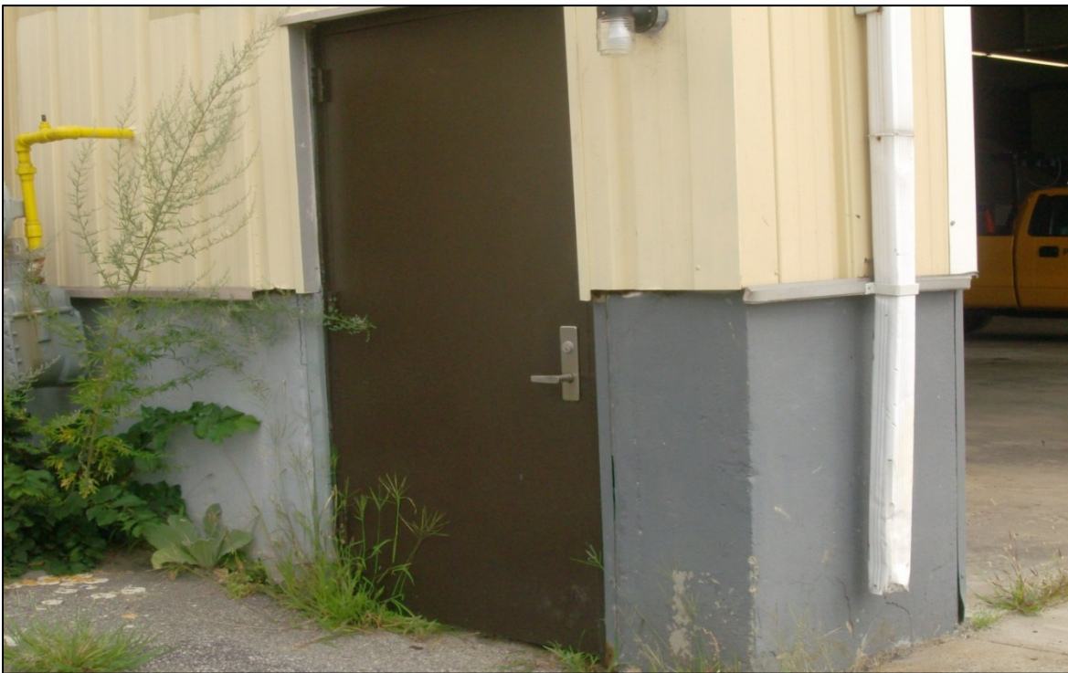
Little used pass door at west side of building.
