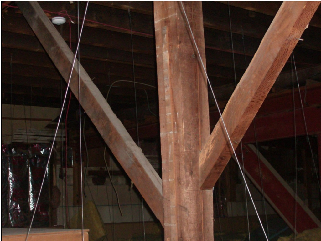
New framing in attic area above Senior Center. Note steel truss in background that was added when second floor walls and floor were removed, and the roof was lowered.
