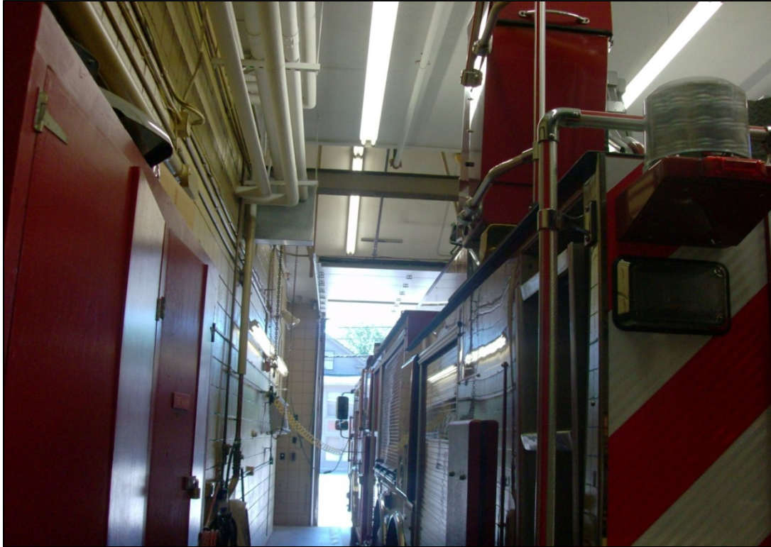
Apparatus bay for Engine 1. Note the lack of clearance.
