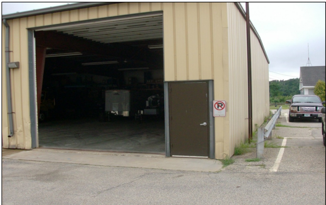
Pass door on west side of building.
