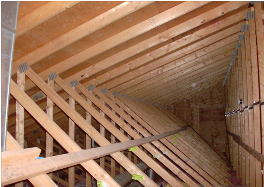
Typical attic space above office.
