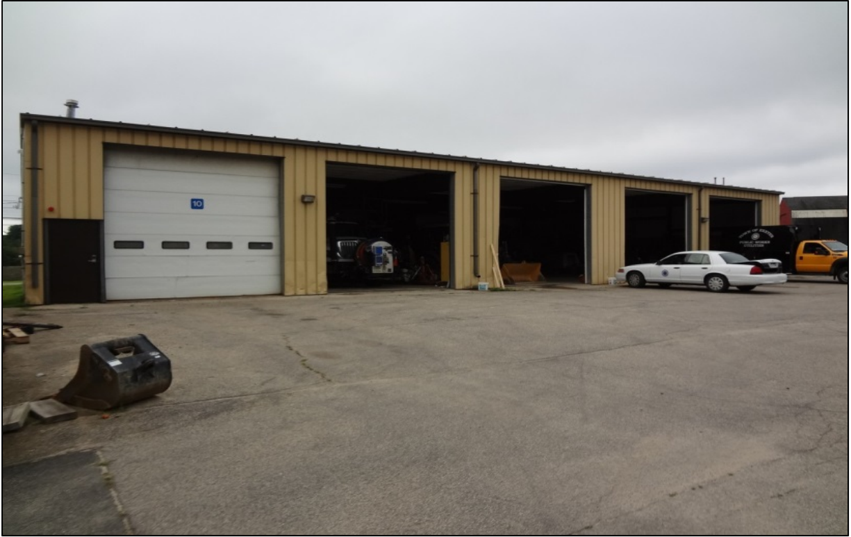
Front of Water Department Garage.
