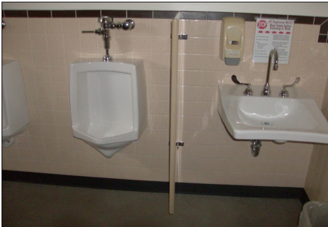
Men's Room with ADA accessible sink.
