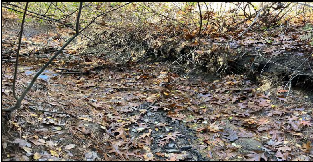
A view of the outlet channel area of Wetland 1B as it meets Parkman Brook in the background.
