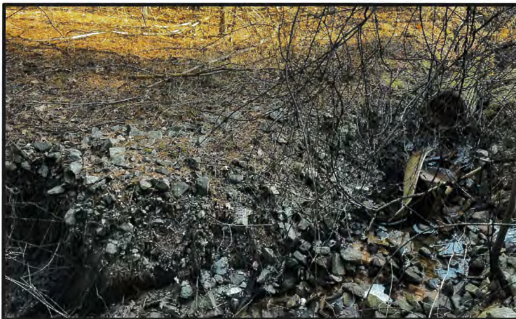
View of the NHDOT Detention Basin Outlet Structure.
