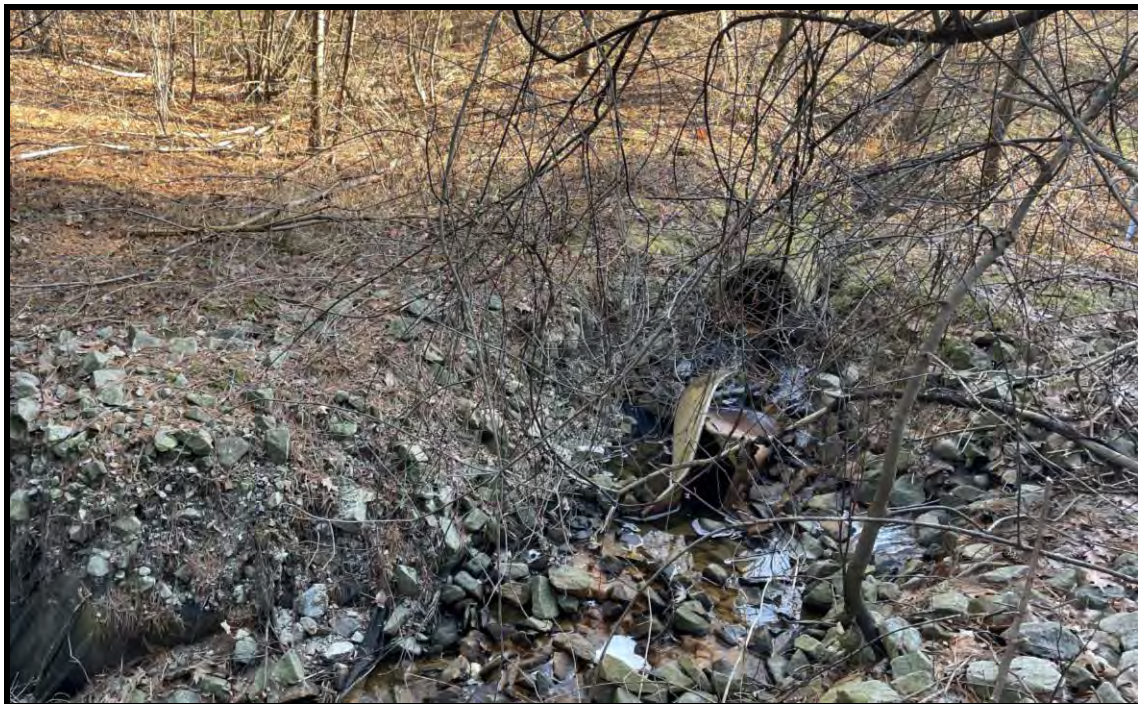
A view of the NHDOT outlet point into the ditched wetland.
