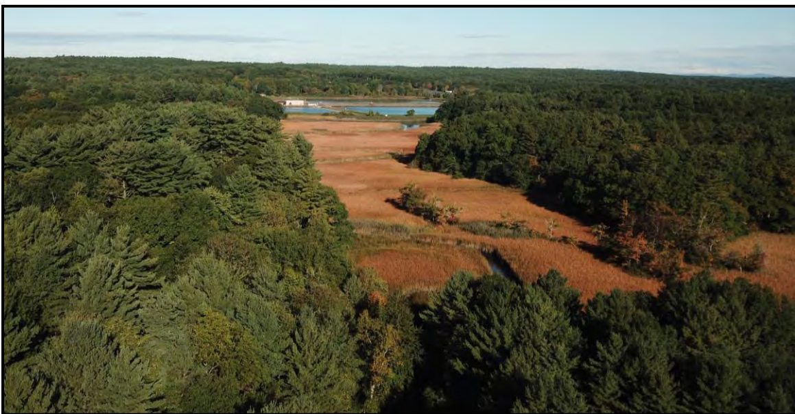
A view looking north at Parkman Brook with the Wastewater Treatment Plant in the background. The project has avoided impacts to the system and has maintained a buffer to the system.
