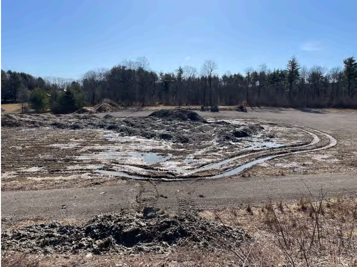
Photo #2. East-facing view of recently-leveled area.
