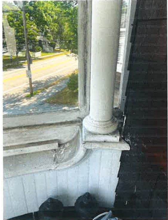
Detail at base of porch column
