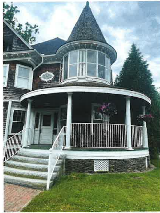
This is how the 2 nd floor tower “porch” has looked for at least the past 25 years.
