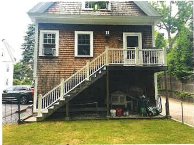
Existing back steps and landing.
