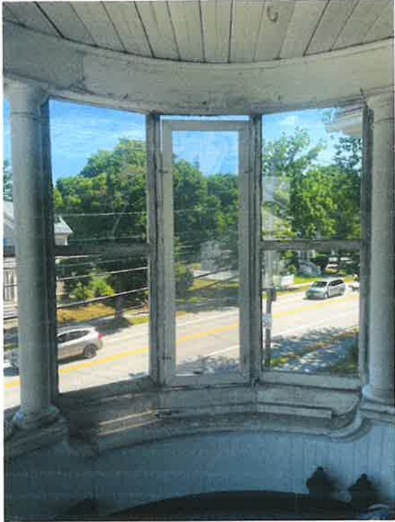
Interior view of round porch
