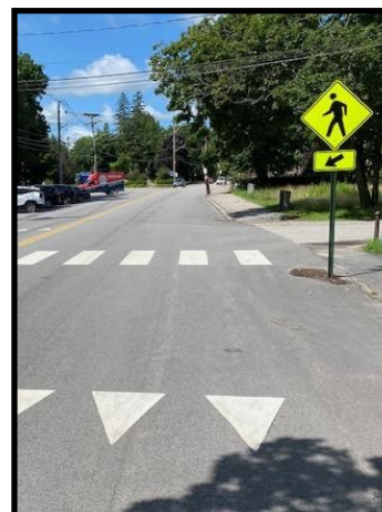
High visibility signs and pavement markings added at crosswalks on Front Street in 2023.
