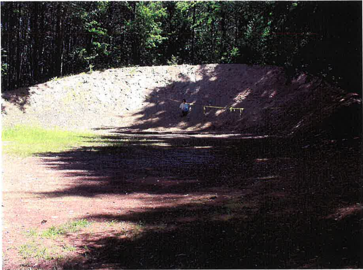
Photo 5 – Existing Rifle Range Soil Berm (Sample Location B-2)
