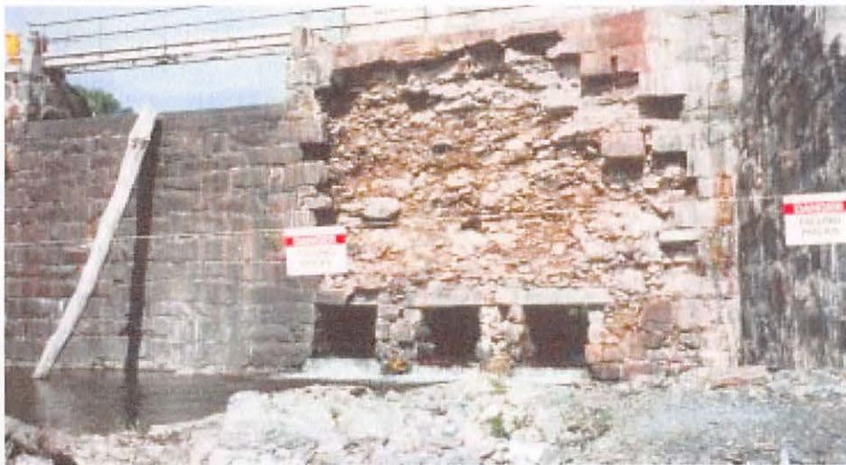
Left: Granite blocks from the Union Gas Dam on Messalonskee Stream in downtown Waterville suddenly collapsed in June 2001. To reduce safety risks, the dam's owner, Florida Power and Light, dismantled a large portion of the dam, allowing the river to run through it.
