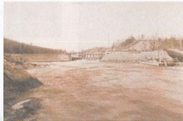
As Maine was settled, dams – such as the Pejepscot Dam (circa 1890) on the Androscoggin River in Topsham – were built on essentially every major river to provide mechanical power to operate mills.
