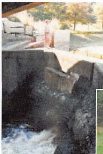
Above: The fishway for the Grist Mill Dam on the Souadabscook Stream no longer functioned.
