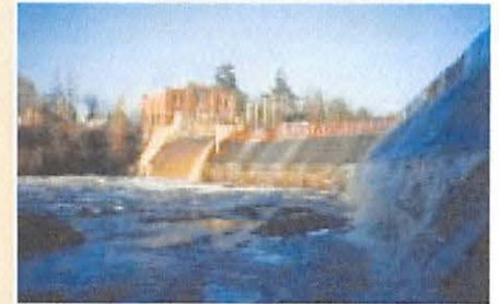
Ft. Halifax Dam
