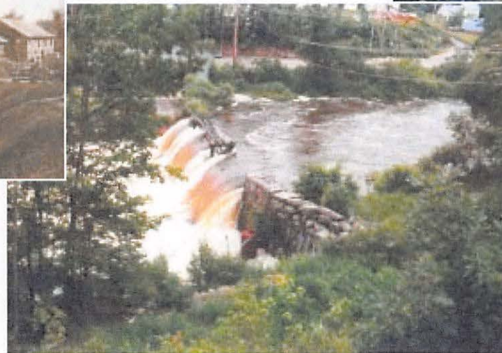
Right: The Gardiner Paperboard Dam, on Cobbosseecontee Stream in Gardiner, is slated to be removed.
