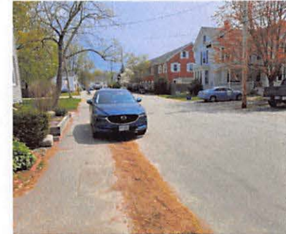
Lack of curbs or delineated parking. Encroachment onto pedestrian sidewalk.
