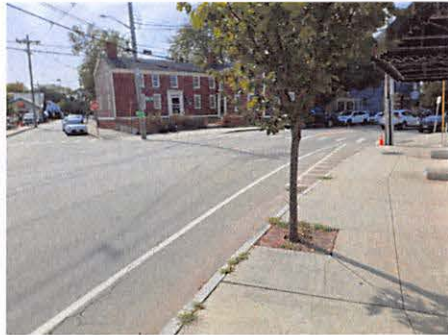
Roadway curvature and limited warnings to drivers
