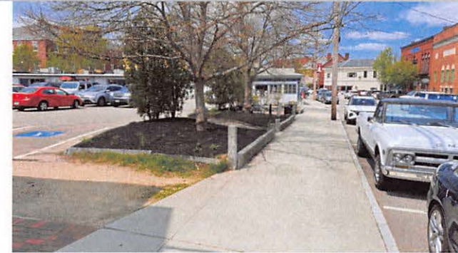
Sign not present at key entrance to Municipal Parking Lot (Source: Stantec Field Inventories)
