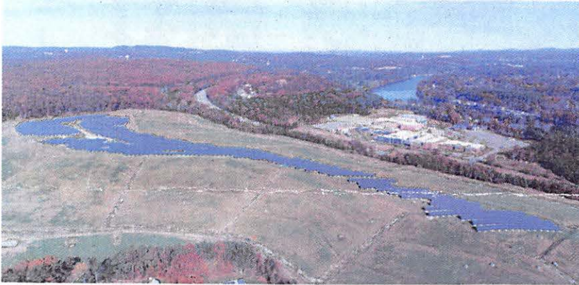
This aerial view shows the large solar array built on Manchester's capped landfill, turning seemingly unusable land into a benefit. Photo Provided by Kearsarge Energy
