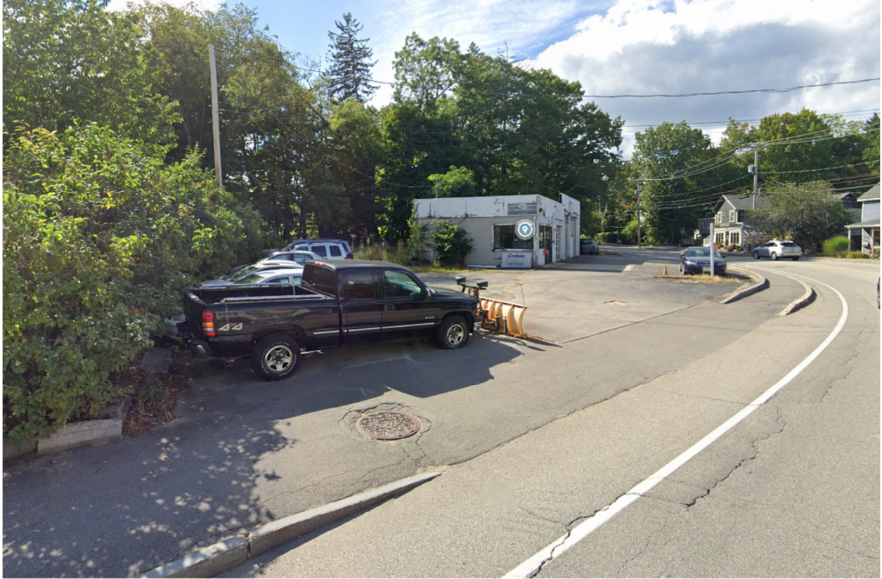
Photo 3 – Northeast property corner. Curb cut will be closed and sidewalk extended.
